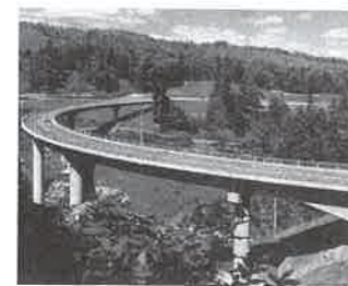
World's first curved bridge by Prof. Noboru Watanabe
